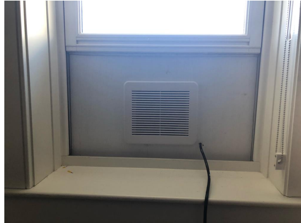
Negative pressure units with HEPA filtration
